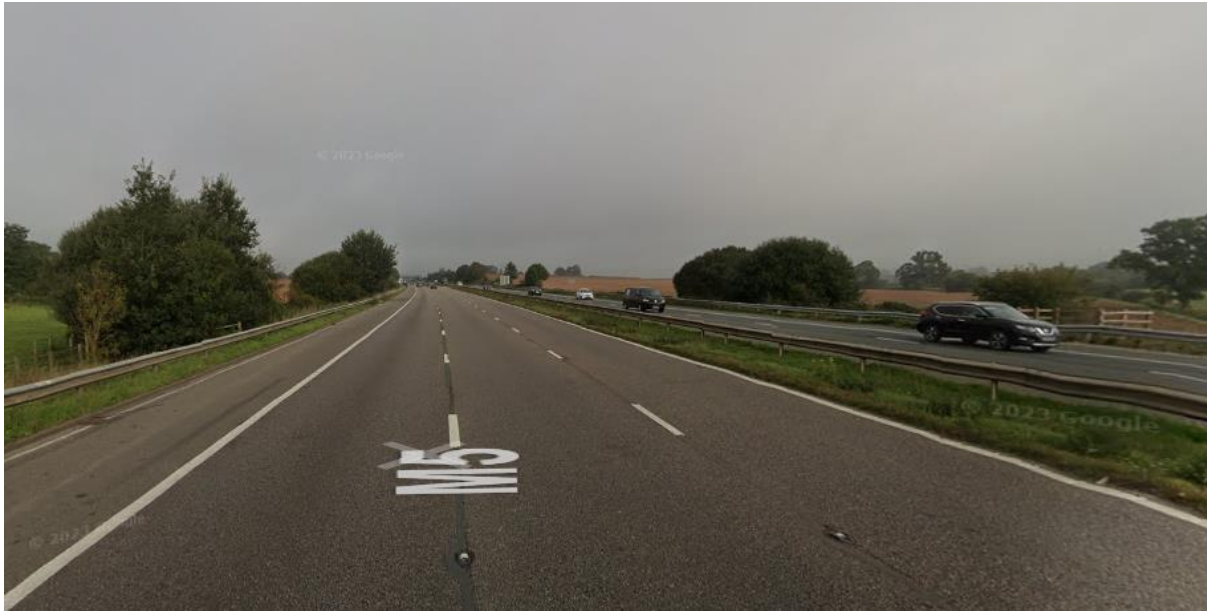
M5 looking north from the south of the site. It can be seen on the right of the road
